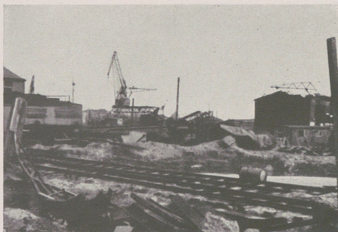
Zniszczenia w porcie są ogromne. The harbour has been bombed thoroughly.
