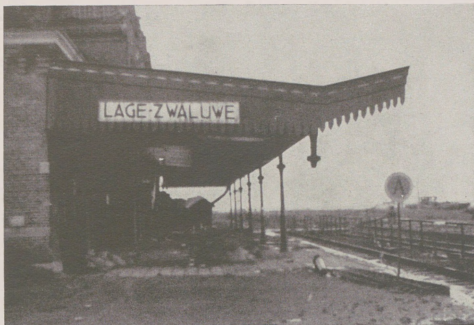
Z rejonu stacji kolejowej tłukły po nas p-pance. Near the railway station we were shelled by anti-tank guns.
