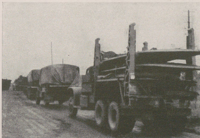
Uszkodzone i zniszczone mosty wymagały wiele materiału do naprawy. Repair of damaged and destroyed bridges took huge quantities of material.
